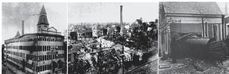
Figure 1. View of the R. B. Grover & Company Shoe Factory before (left) and after (middle and right) the boiler explosion on March 20, 1905, that killed 58 persons and injured 117, (USGenWeb, 2011, Ellenberger et al., 2004).
