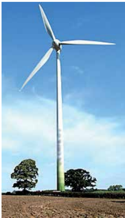
Figure 2.9 Commercial wind turbine with horizontal axis.
