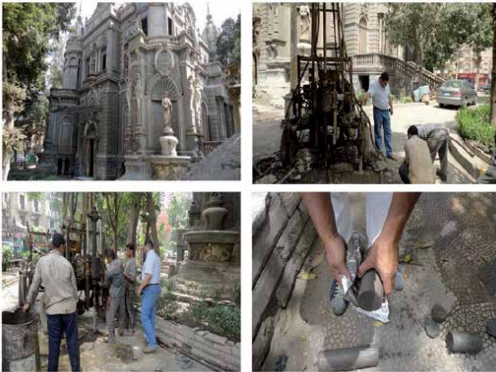
Figure 5. El- Sakakini palace and the Geotechnical investigations.
