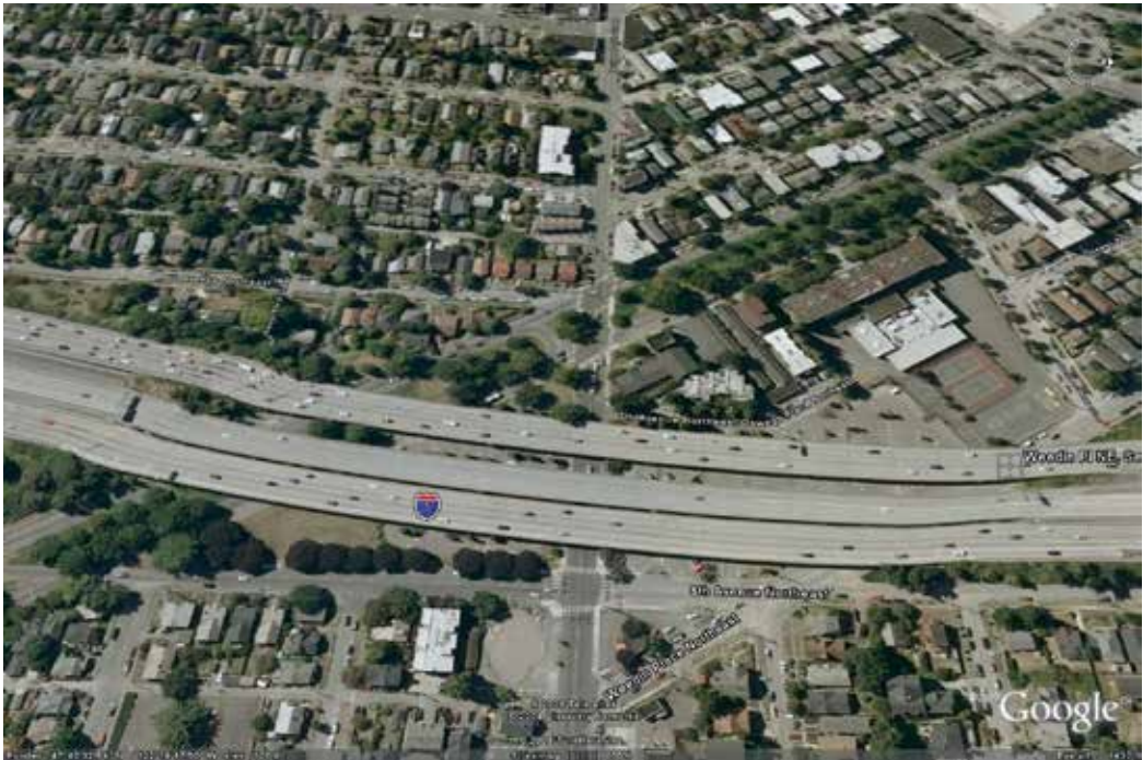
Figure 1. Aerial view of the North Bound bridge
