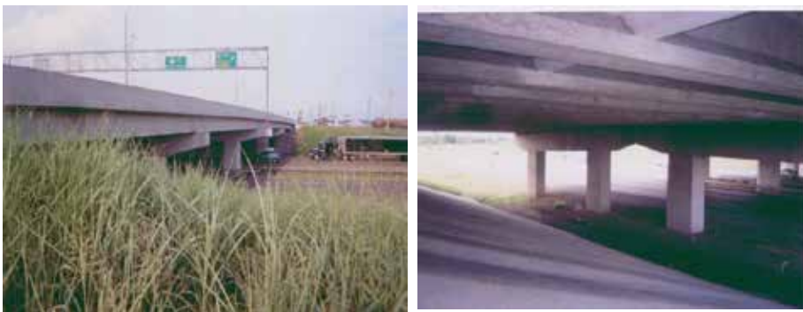
Figure 4. Bridge carrying MS 302 over Interstate highway I 55; (left) looking toward Southaven, MS, a fast growing city forming part of the metropolitan area of the City of Memphis; (right) view of the intermediate bents and girders of the two closely spaced bridges
