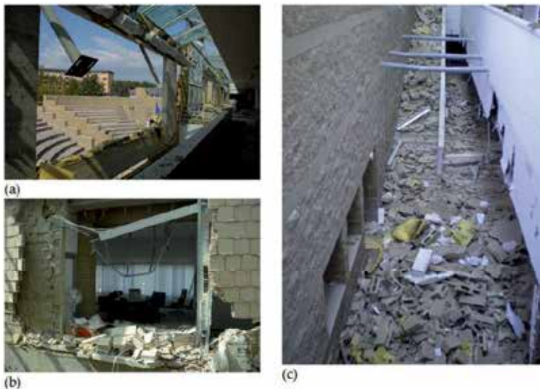
Figure 3. Damages caused by 2009 earthquake to the Edifice A: a) internal view of the main facade, b) internal partitioning walls c) heavy bricks fallen down inside the building from the facade.
