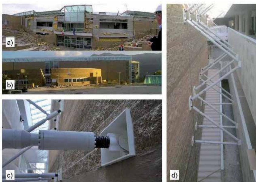
Figure 9. Reconstruction at Edifice A: a) damage scenario involving the facade, b) reconstruction of the facade, c) close view of the installed device, d) dissipative truss structures.
