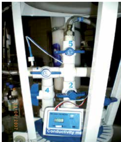
Fig. 9. Photography of a flow distributing and conductivity measuring part of the pilot one body multi stage multi cell water deionization filtration device
