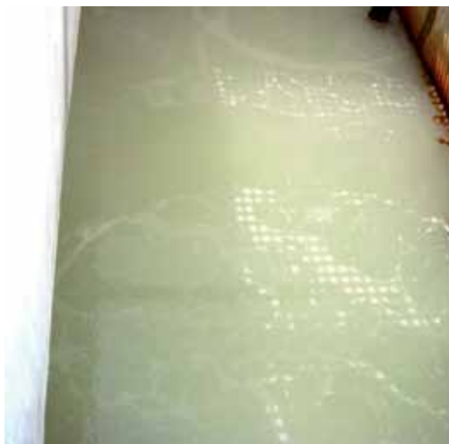
Fig. 30. White water formation (Spidflow™)
