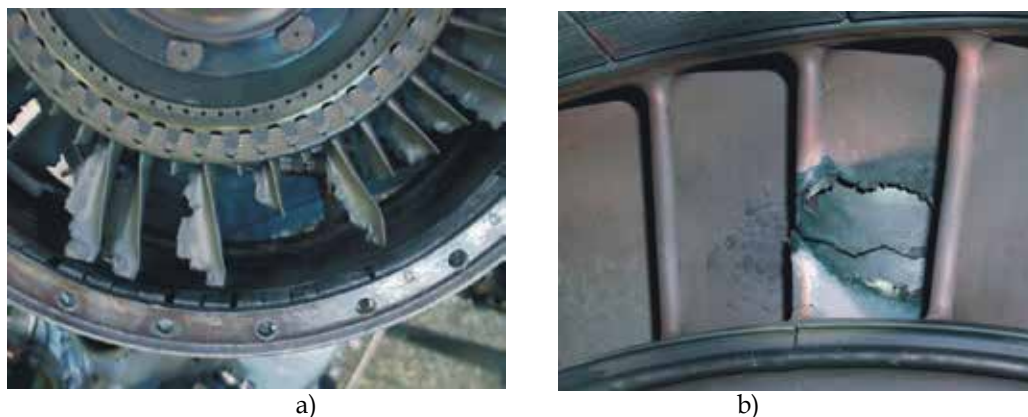
Fig. 8. Characteristic forms of failures to gas turbine caused by long-lasting excessive temperature of exhaust gases (Reports, 2000-2010): a) – burn-through of turbine rotor blades, b) – melting of a nozzle vane
