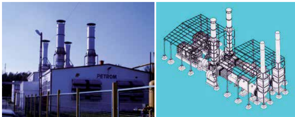
Fig. 1. 2xST 18 Cogenerative Power Plant view (left) and gear placement (right)
