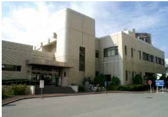
Fig. 13. Yamaguchi University library building
