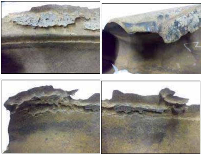
Figure 7. Wall thinning and pits at 5 – 7 o'clock position of downstream part.
