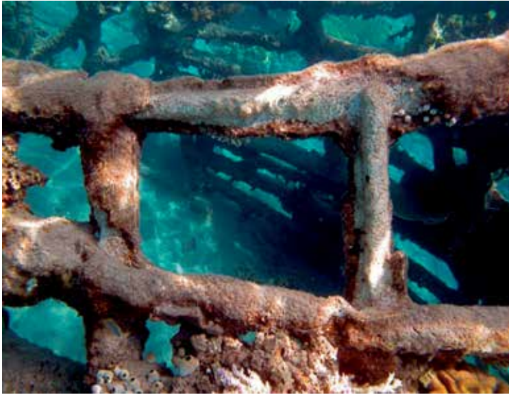
Figure 4. Self repair of Biorock damaged by big boat impact. Time series photographs by Rani Morrow-Wuigk. This structure was installed in June 2000. Note there is no rust on the steel after nearly 11 years in seawater.
