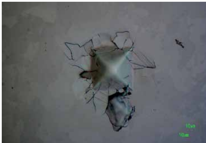
Figure 9. Brittle two-phase regions on the surface leading to indentation cracking.
