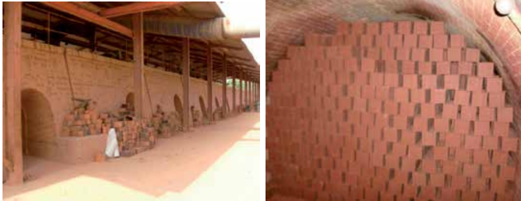
Figure 8. Tunnel kiln and its inner chamber
