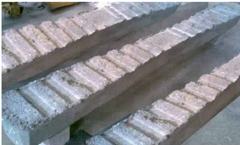
Fig. 14. The bottom of frictional concrete sleeper
