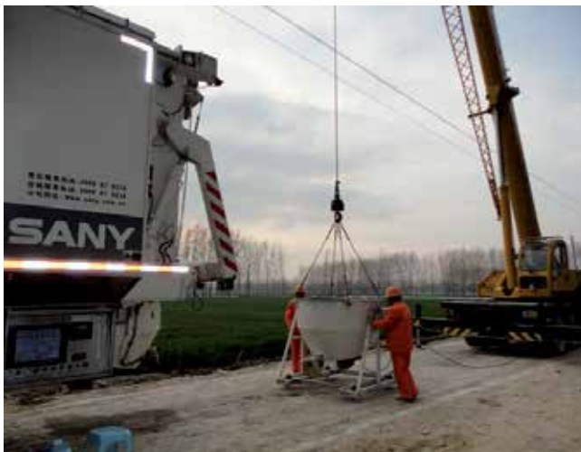
(a)Transportation of CA mortar
