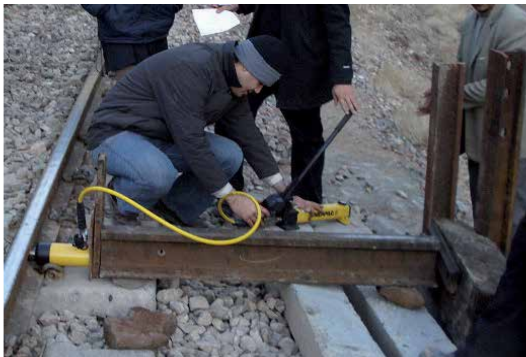
Fig. 15. Installation of the hydraulic jack
