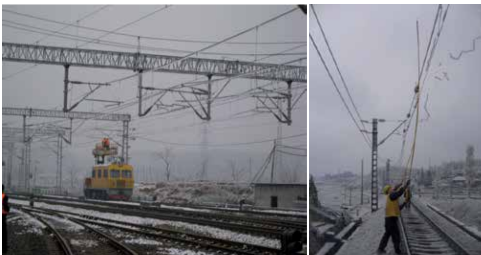
Fig. 1-1. Manual de-icing on overhead contact wires
