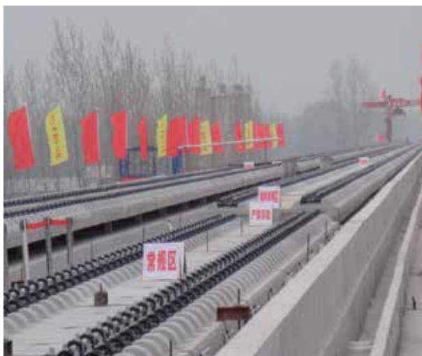
Fig. 31. Preparation before grouting
