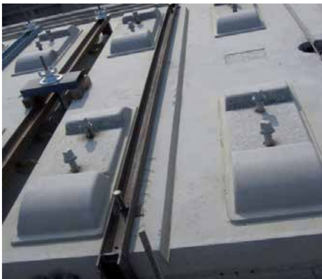
Fig. 33. Tight the slab track
