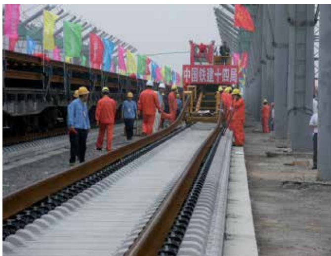
Fig. 40. Railway track laying
