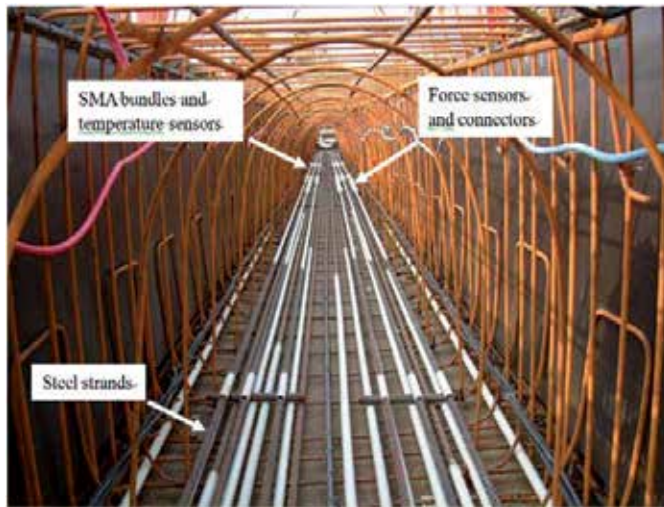
Figure 32. Framework of steel reinforcement with stretched SMA bundles
