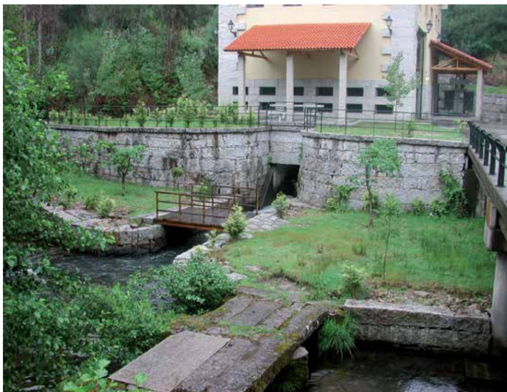
Fig. 2. Central power station of the DevaPO River (Pontevedra, NW Spain).
