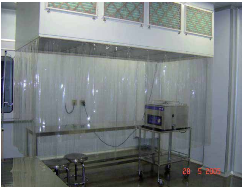
Illustration 03. Classified processing room (100 particles/m 3 air: Class 100/ISO 5; HEPA Filters 99.9 %)
