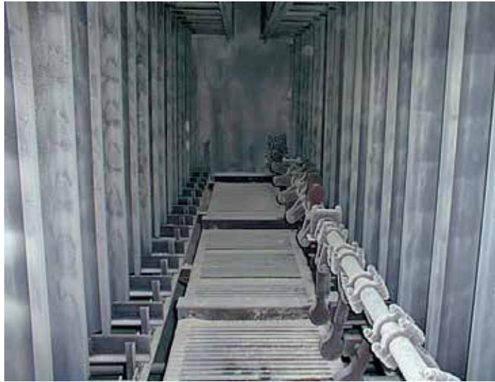
Fig. 2. Inner part of the ESP.
