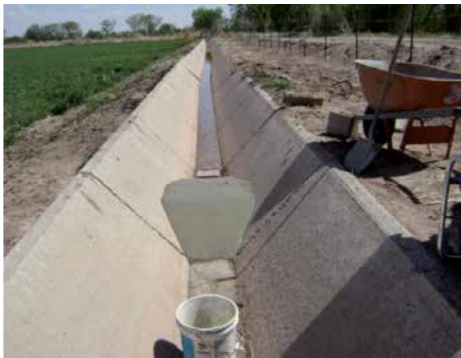
Fig. 5. Completed Broad Crested Weir for Field 3
