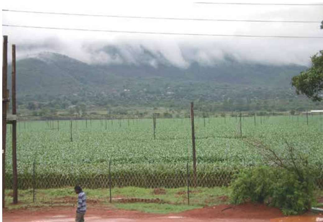
Fig. 3. Revitalisation of Tshiombo Block 1A replaced the secondary canals and concrete furrows that conveyed water to the edge of individual farmers' fields with a centrally operated floppy sprinkler system that covers the entire hydraulic unit
