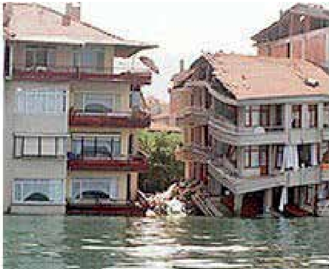
Fig. 8b. An example of liquefaction in TURKEY after 1999 Marmara Earthquake. It is taken from http://www.kenthaber.com/marmara/kocaeli/Haber/Genel/Normal/depremde-yikilan-konuta-imza-atti/3d13f1c8-4158-4ce1-b380-13e53de1be21 . Photographer is unknown.
