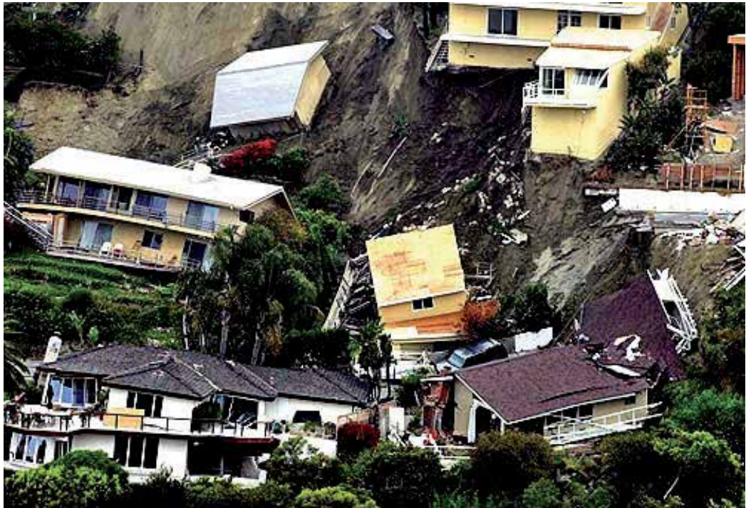
Fig. 7b. An example of landslide in Laguna Beach, Bluebird Canyon, California . It was developed in steep and high slope. It is taken from USGS website (US Geological Survey). Photographer is Jim Budak.
