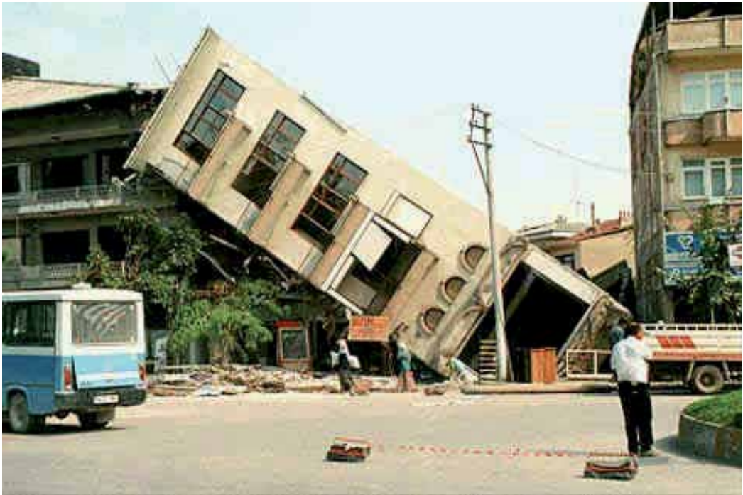
Fig. 8a. An example of liquefaction in TURKEY after 1999 Marmara Earthquake. It is taken from http://www.el-aziz.net/img4381.htm . Photographer is unknown.
