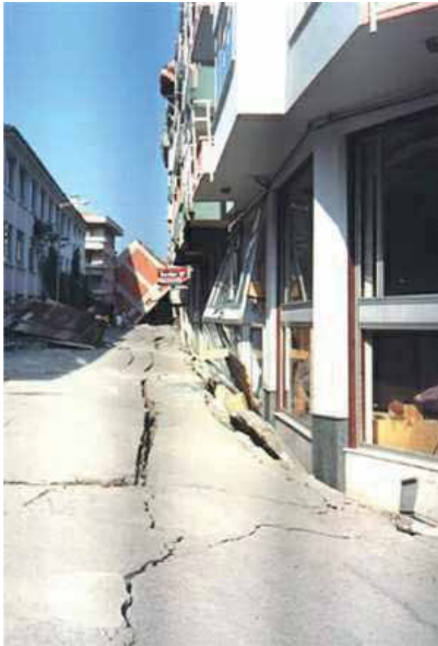
Fig. 4. An example of loose soil in Adapazarı after 1999 Marmara earthquake. It is taken from http://avnidincer.8m.com/depfoto.html . Photographer is Eşref Yalçınkaya.
