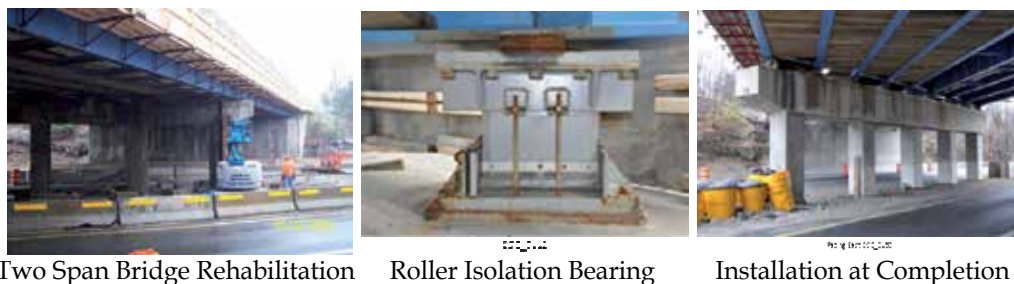
Fig. 5.3. Bridge Rehabilitation in Rhode Island
