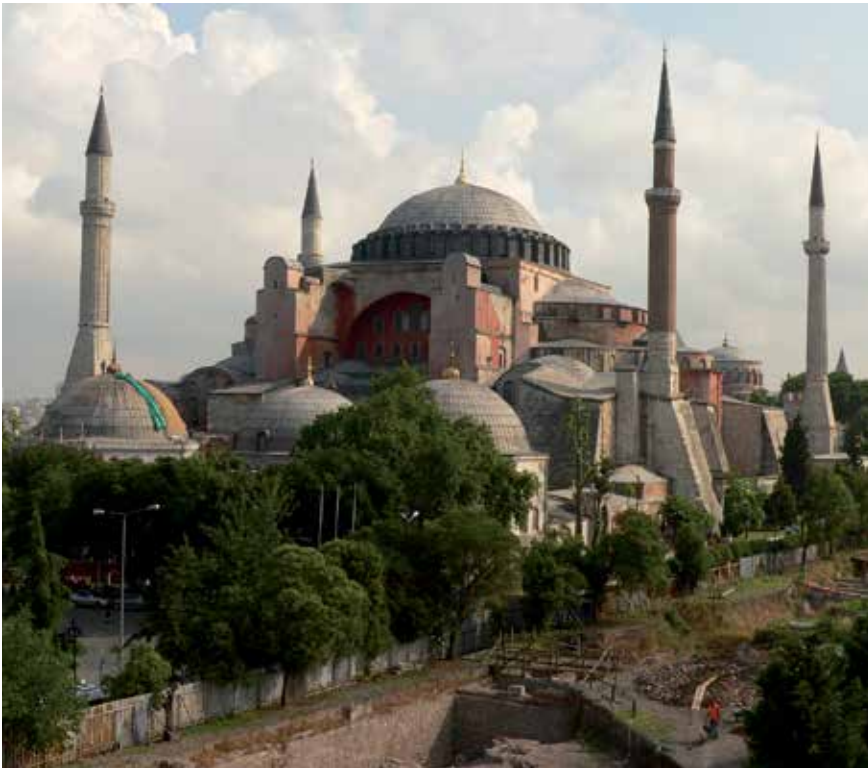
Fig. 1. Hagia Sophia is strengthened with external buttress type walls by Sinan in 1573.
