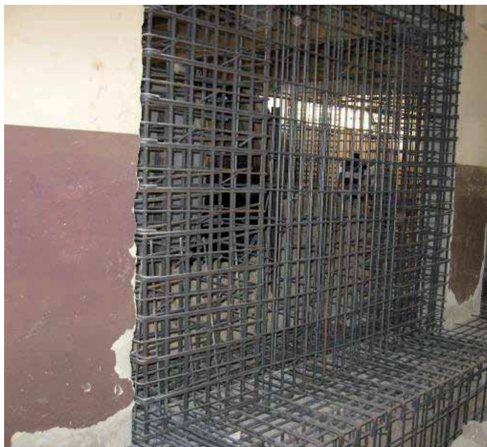
Fig. 3. Infill wall application in an RC building
