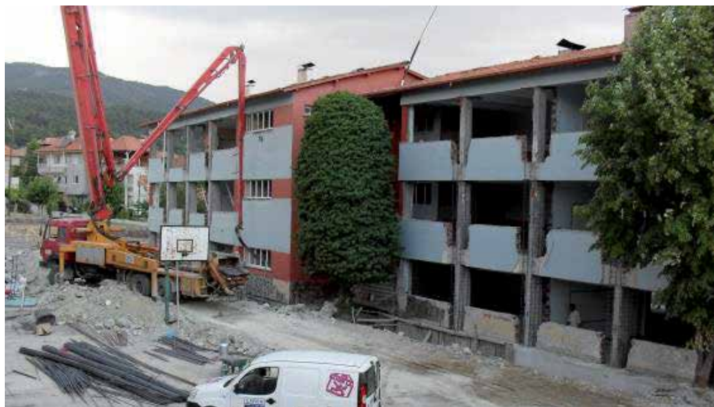
Fig. 12. An RC jacketing application (Photo by Ahmet Sarışın)
