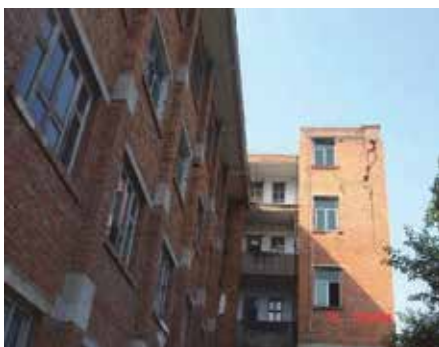
Fig. 6. Severe damage of masonry buildings with plan irregularity
