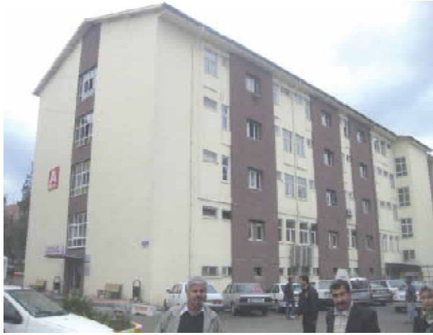
Fig. 8. An external shear wall strengthened building
