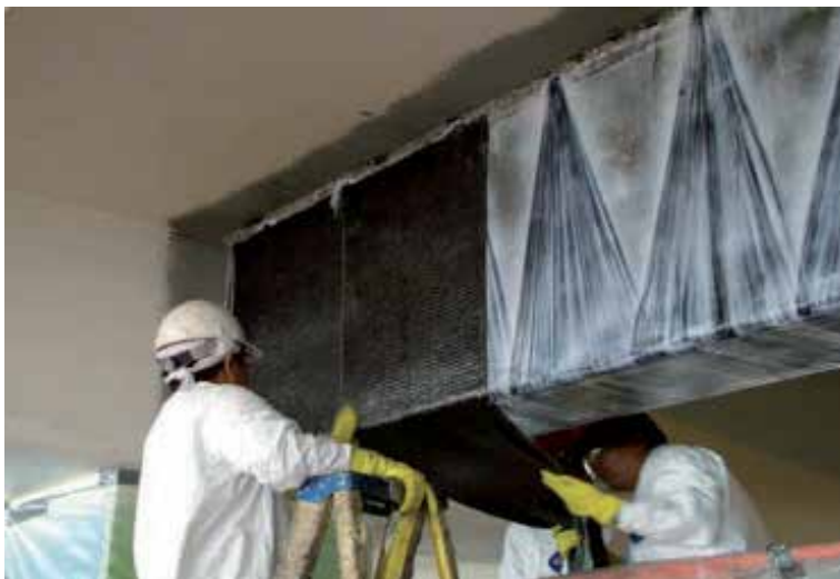
Fig. 14. FRP confinement of a beam (reprinted with the permission of FYFE Europe)
