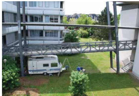
Fig. 13. North view of the bridge subjected to monitoring.
