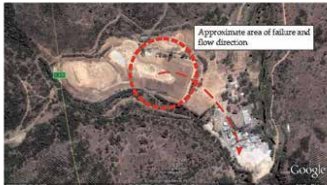
Fig. 23. Bird's-eye View of Las Palmas Tailings Impoundment Prior to Failure. (GEER 2010)
