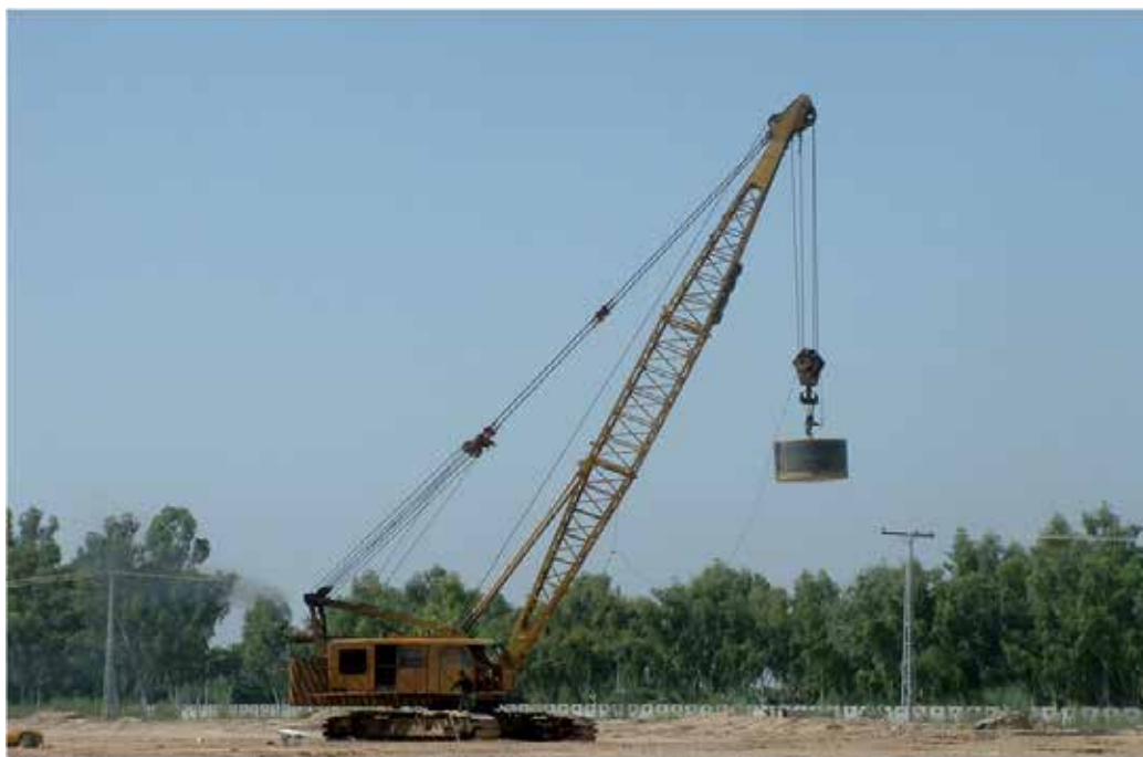
Fig. 3. Dynamic Compaction Equipment (heavy crane, tamper, release mechanism) and process
