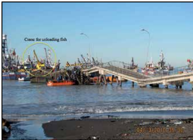
Fig. 22. Distorted Fish-Unloading Concrete Pier at Coronel Port, Chile. (TCLEE 2010)
