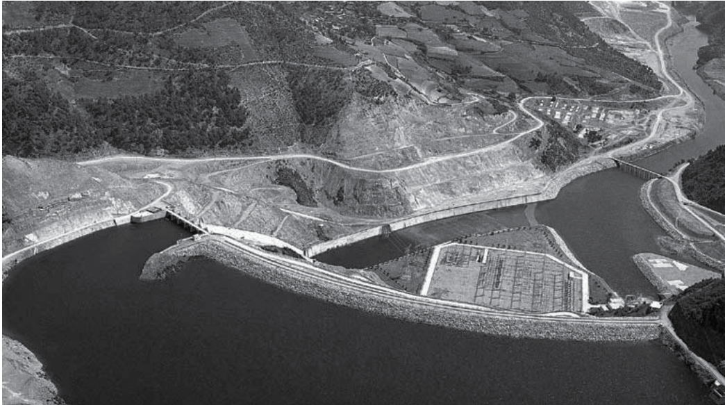
Fig. 5. View of the Altinkaya dam
