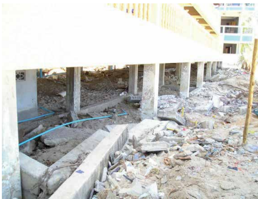
Fig. 42. Close-up of Fig. 41, Showing Inter-connected Grade Beams and Columns.
