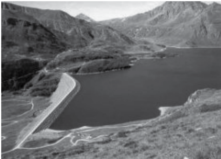
Fig. 13. View of the Boztepe dam
