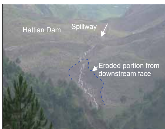
Fig. 7. Front view of the Hattian landslide mass, showing the downstream face erosion.
