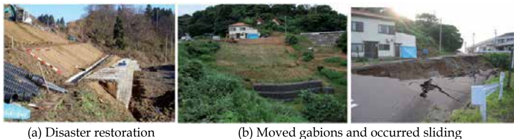
Photo 11. Application of large-scaled gabion at present
