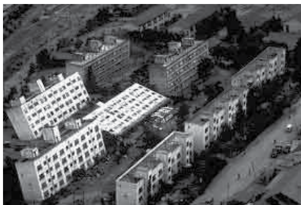
Fig. 1. Apartment buildings at Kawagishi-Cho, Niigata, Japan, tipped after the foundation soil liquefied during the 1964 earthquake.
