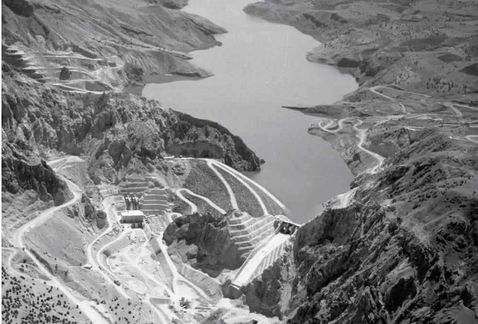
Fig. 7. View of the Kilickaya dam
