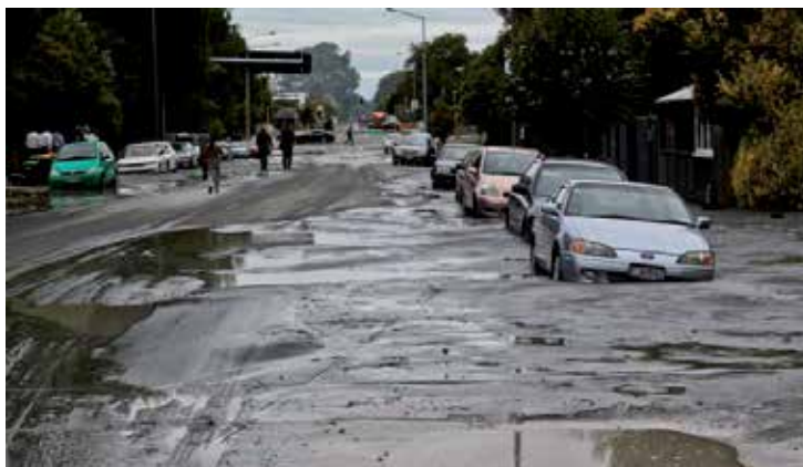
Fig. 26. Liquefied Sand Deposited on Street, 2011. http://otilya.com/view/ News/Asia-Pacific/New-Zealand
