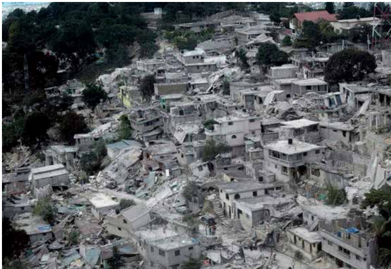
Fig. 19. Damaged Buildings Located on Hill Slope. http://www.worldcatastrophe.com
