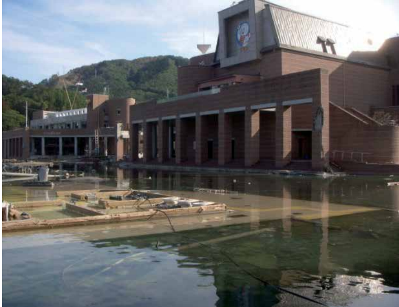
Fig. 33. Waterfront Buildings in Onagawa, Japan Inundated by Tidal Water Due to Earthquake Subsidence. http://tectonics.caltech.edu/slip_history/2011_taiheiyo-oki/index.html
