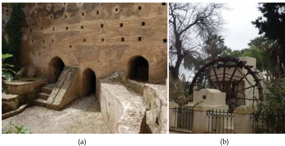
Fig. 5. a) Water distributor, Fes b) Noria from which the water flowed to the distributor
