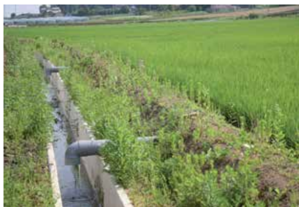
Photo 5. Drainage canal separated from dual-purpose canal, irrigation and drainage
