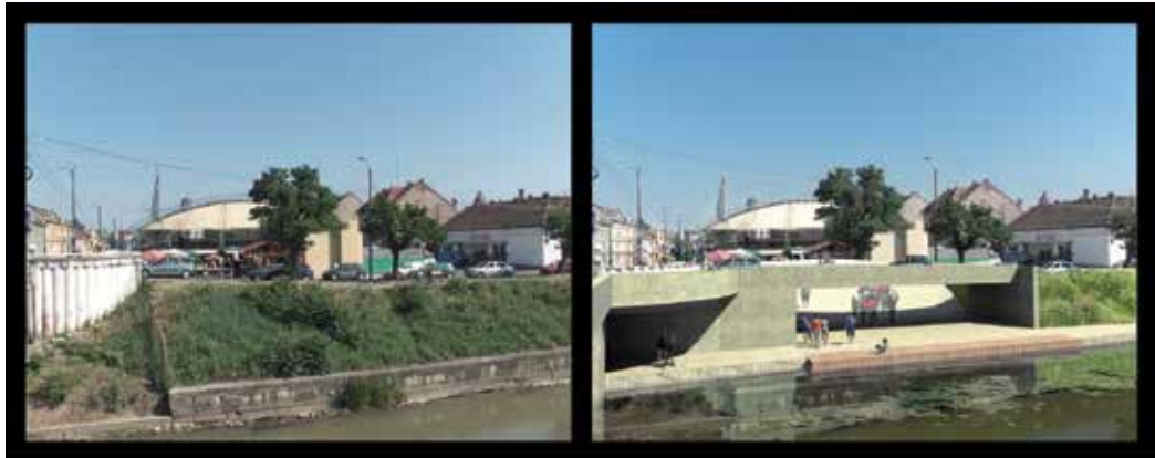
Fig. 18. The riverside of the Bega Canal – current situation and proposal from disertation papers within the Master of Urbanism and Territorial Planning, coordinated by The Reseach Group for a Sustainable Territorial Development
