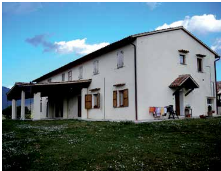
Fig. 1. External view of the building
