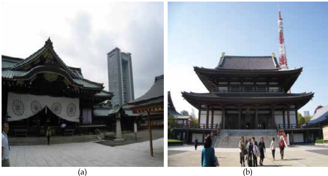
Fig. 1. (a) A Japanese historical Shinto shrine and a new tall glassy building behind, (b) A Japanese historical Buddhist temple and a tall broadcasting tower behind
