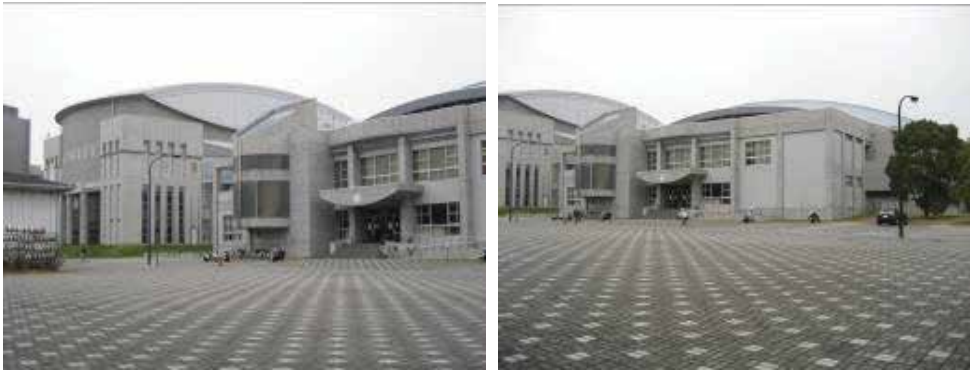
Fig. 6. Convention Center (left) and Gymnastic Hall (right) of Osaka University
