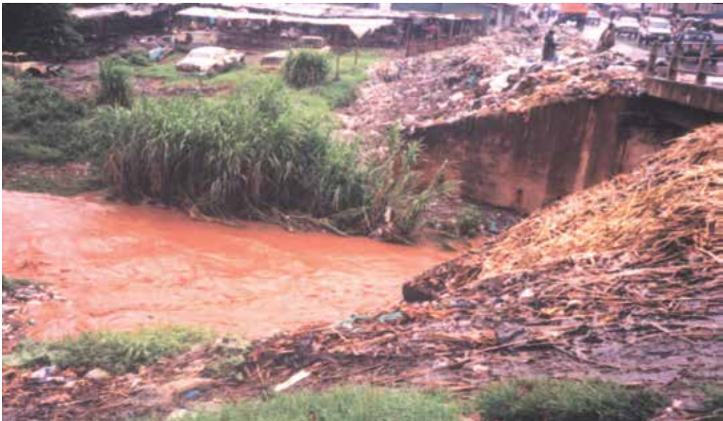
Photo 1. Gikomba-Shauri Moyo Bridge D/S Gikomba open-air market-solid wastes, Car shells and Jua Kali garages in the foreground.
