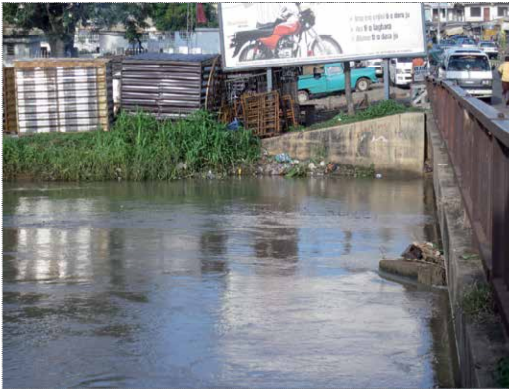
Fig. 4. Metal works along river bank
