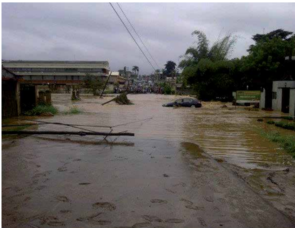
Fig. 1. A picture showing the devastating effects of the flood incidence of 25 th August 2011 in parts of Ibadan city
