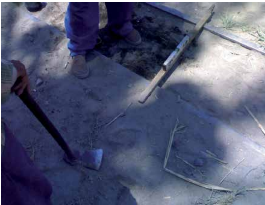
Fig. 22. Balancing the level of the rail track
