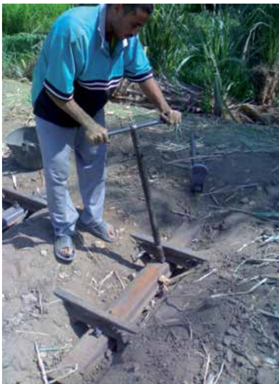
Fig. 21. Replacing the corroded steel sleepers of the rail track
