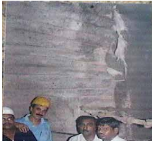
Fig. 5(b). Pier nose wall after pre-split blasting
