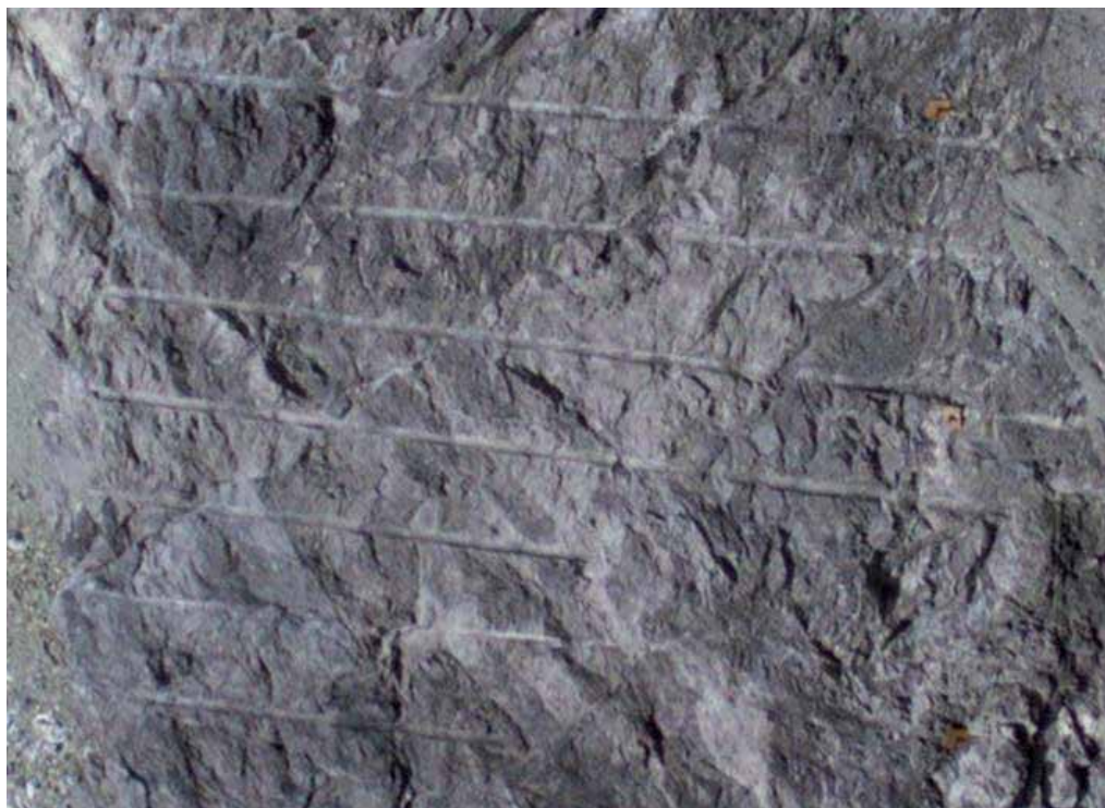
Fig. 7. Improved blast performance of smooth blasting in the form of smooth profile at KHEPP
