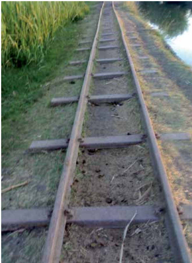
Fig. 5. A balastless narrow railway expanded on a bank of an irrigation channel
