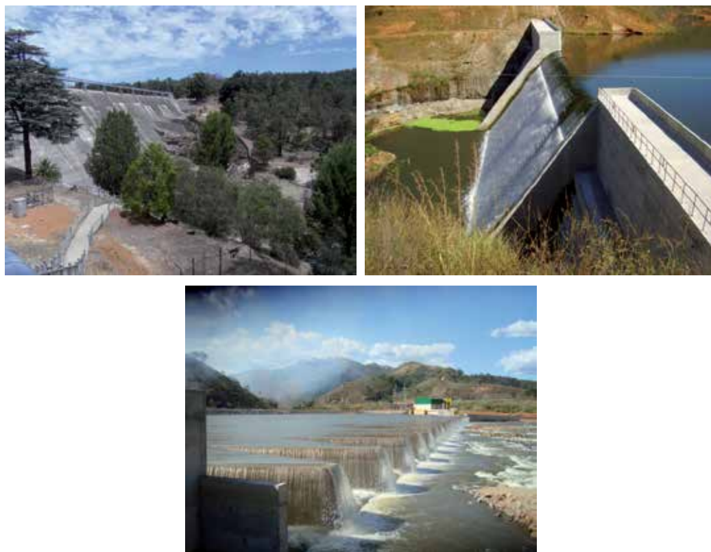
Fig. 1. Illustration of dam structures: a) Traditional smooth chute, b) Flow over a stepped chute, c) Labyrinth (Picture acknowledgements: Fig.1a: Stuart Longley; Fig.1b and Fig.1c: Engevix Company).
