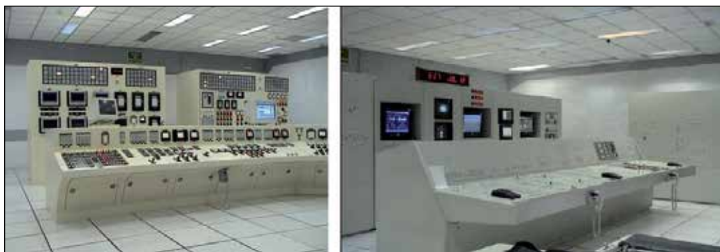
Fig. 2. Control board simulators.
