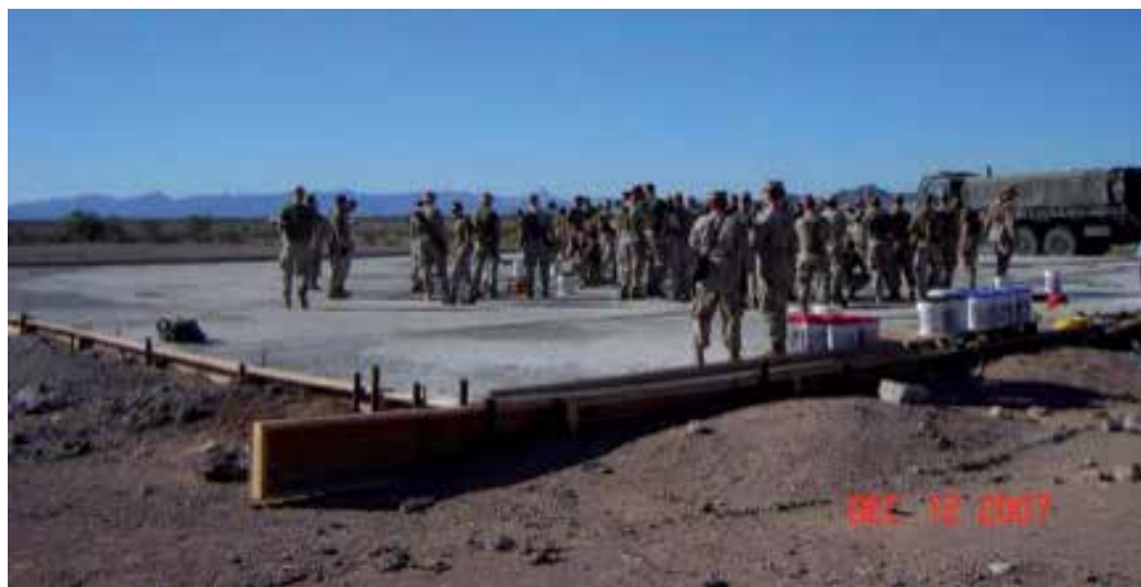
Fig. 5. Marine Corps Engineers training for fast track construction and repair prior to deployment. Marine Corps Base Concrete Installation, (James K. Hicks, et. al., 2009).
