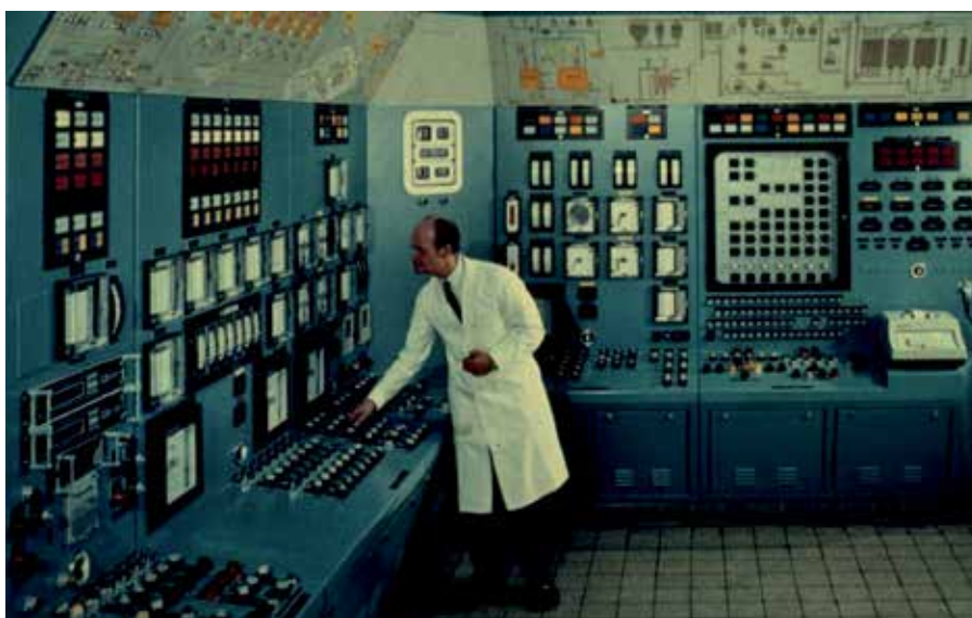
Fig. 2. Wall panels with a good overview and full interaction.
