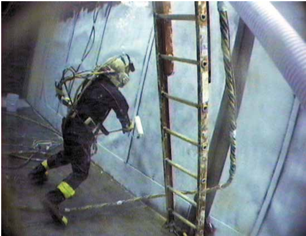
Fig. 2. Special two hose roller system used for wall coating at the MTR pool.
