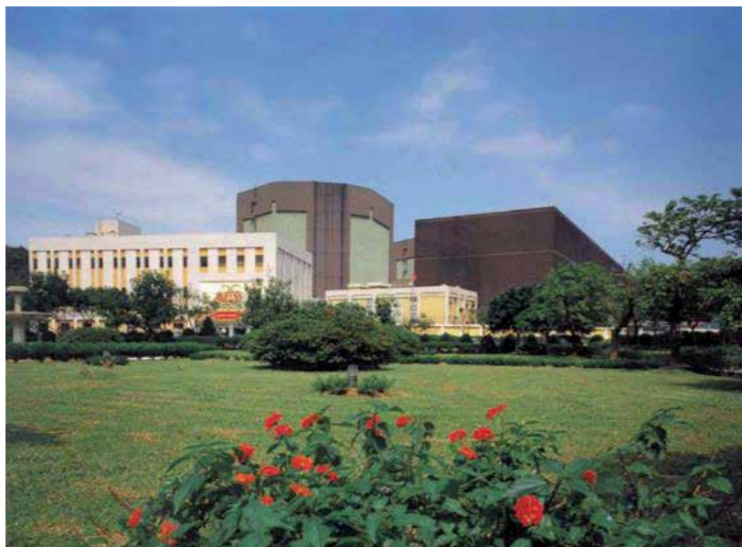
(2) Kuosheng nuclear power plant (From http://www.aesieap0910.org/ )
