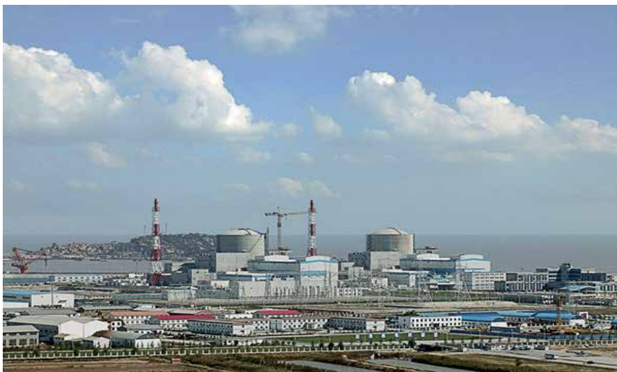
D: Tianwan Nuclear Power Plant in China (From http://www.heneng.net.cn/ )
