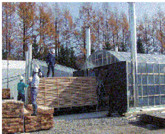
Photo 1. A Fully Passive Solar Lumber Drying House Loading Larch Lumber (2x4 material); (South-North model)
