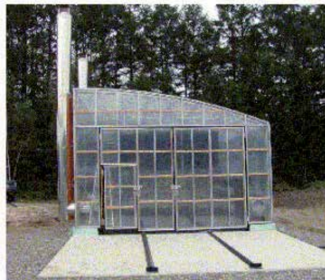
Photo 2. Front View of A Fully Passive-type Solar Lumber Drying House; (East-West model)
