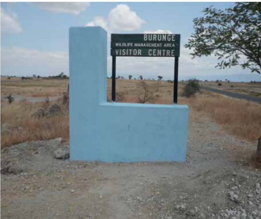
Fig. 1. Burunge Tourist Centre under construction. Photo by Gerson Mollel, 2011
