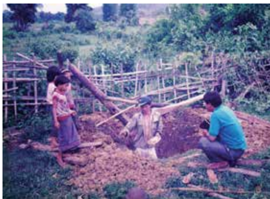
Picture 3. Making of pit for toilet
