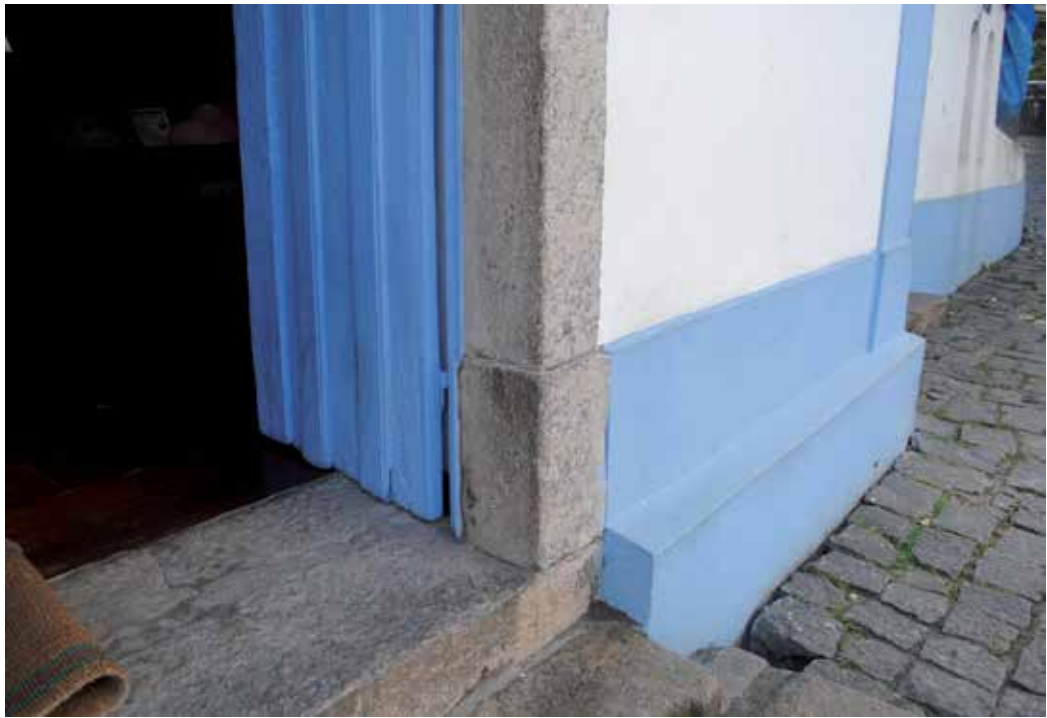
Fig. 9. Detail of a doorframe constructed in the 17th century in Rio de Janeiro.
