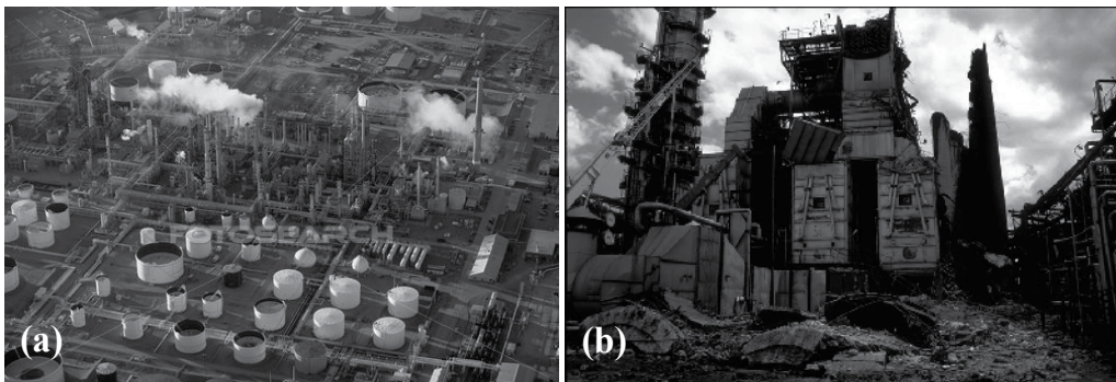
Fig. 1. (a) Areal view of a refinery, (b) Damage in a process furnace (Izmit, 1999).
