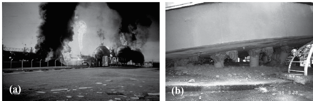
Fig. 5. (a) Butane sphere fire (K. Kounty, 1952), (b) Collapse of LNG tanks (Itzmit, 1999).
