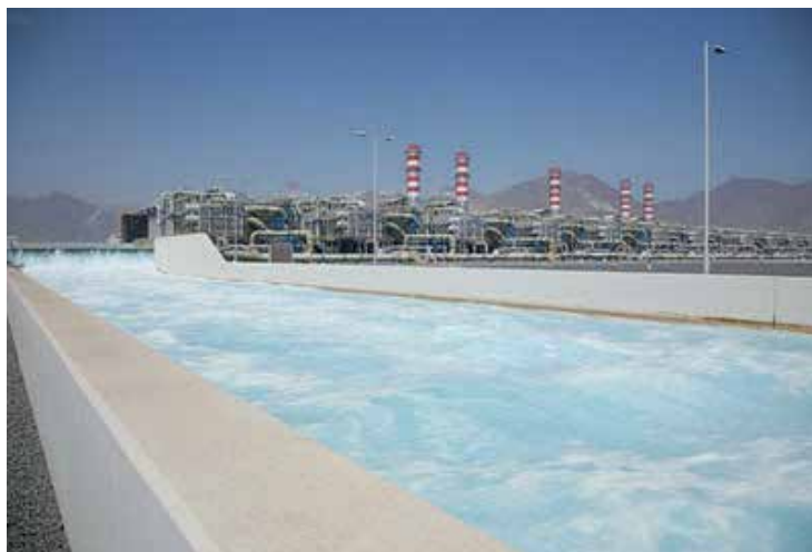
Fig. 6. Fujairah desalination plant in United Arab Emirates, from http://fujairahinfocus.blogspot.com/2011/10/fujairah-power-and-desalination-plant.html
