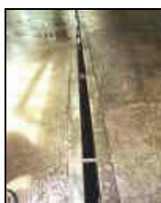
Photo 1. Dirty water generation: wash down high volume low pressure hose and drainage channel for speeding up washing after milking (Source: www.teagasc.ie )
