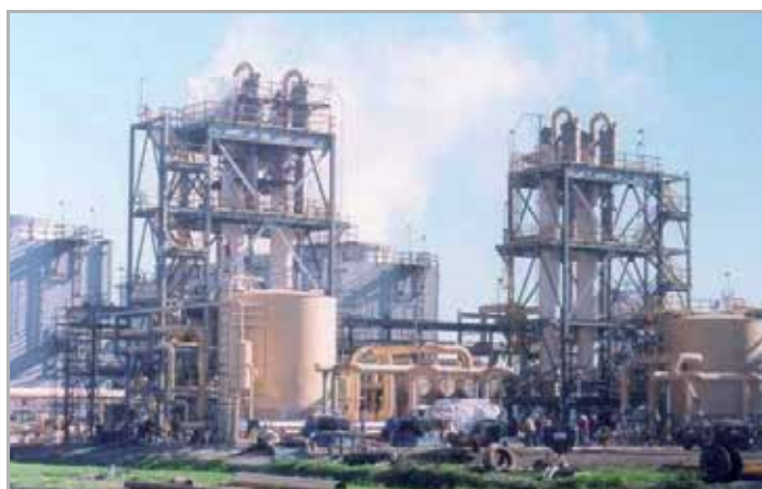
Fig. 14. Installation of 4 600 m 2 self-cleaning surface replacing 24 000 m 2 conventional surface.
