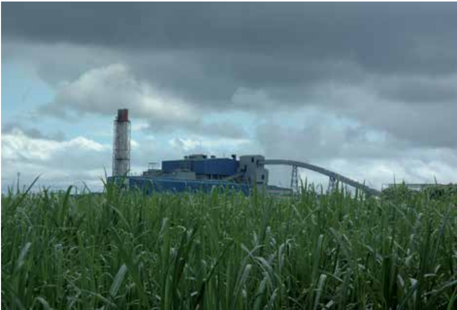
Fig. 24. Sugarcane burning biomass power plant, Mauritius
