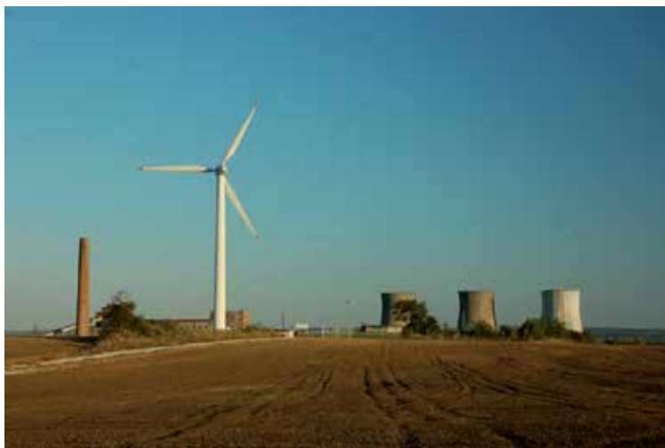
Fig. 22. Wind turbine in Inota, Hungary. In the background is an old coal fired plant.
