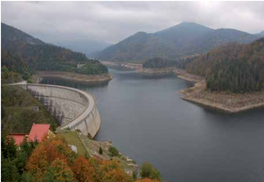
Fig. 26. Hydro reservoir in Bihor Mountains, Romania
