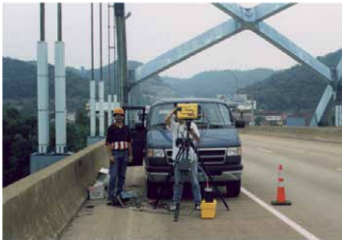
Fig. 14. Cable Vibration Measurements from the Bridge Deck [41] (Chen et al. 2005)
