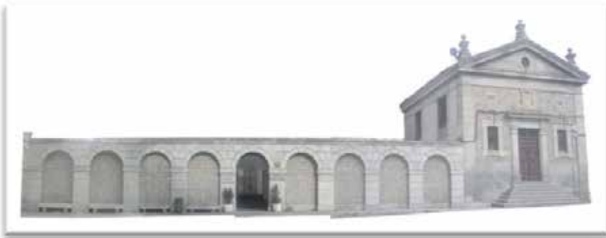
Fig. 12. Final image of the façade obtained from three photographs.
