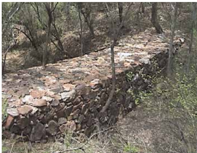
Fig. 3. Retenidas for runoff control in La Labor
