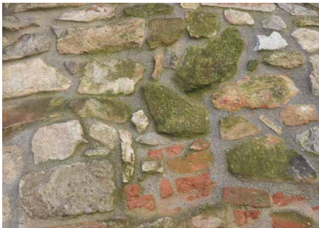
Fig. 2. Different phototrophic colonization in accordance with moisture availability in a stone microhabitat (wall from historical center of Gavorrano, Italy)
