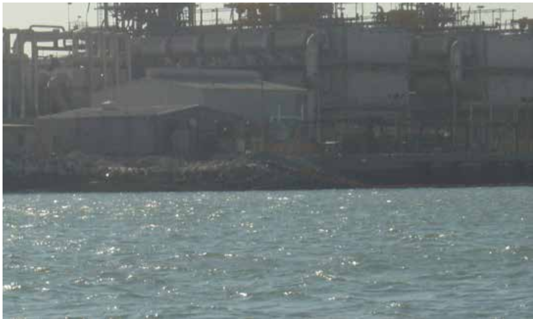
Fig. 4. Sitra Power and Water Station.
