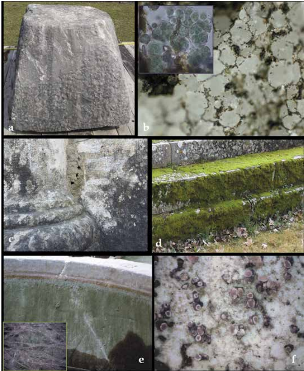
Fig. 7. Different patterns of biological growths found on monumental stones: (a) homogenous black crust with a detail (b) of intergranular development of threadlike microcolonies containing cyanobacteria and black fungi, as revealed by microscopic insight, Carrara Marble Museum, Italy; (c) heterogenous lichenic black crust with a wasp nest on a limestone tomb, Trespiano monumental cemetery; (d) bryophyte extended carpets, Fiesole archeological site, Italy; (e) fibrous microbial mat with a filamentous diatom ( Melosira sp.) as a dominant species, Lindaraja Fountain from Alhambra complex, Granada (Spain); (f) micropits containing the apotheci of an endolithic lichen, Trespiano monumental cemetery
