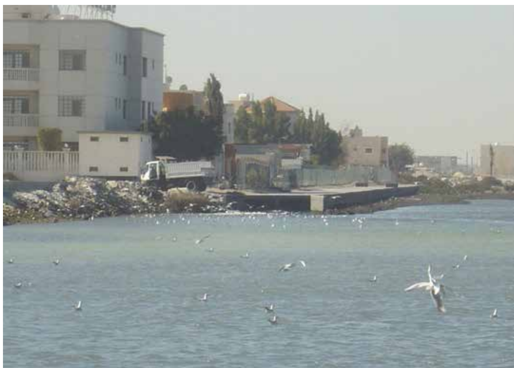
Fig. 3. The outfall of Tubli Water Pollution Control Centre, the main sewage treatment plant in Bahrain.
