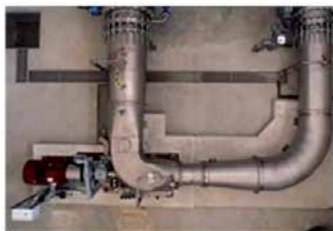
Fig. 7 and Photo 34. Setting of a Kaplan turbine as a bypass of an existing valve in a drinking water network (case study Poggio Cuculo).
