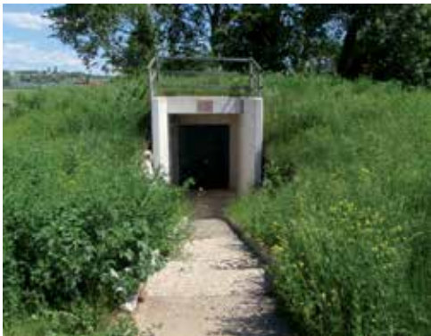
Photo 3. Armyary: the power house.
