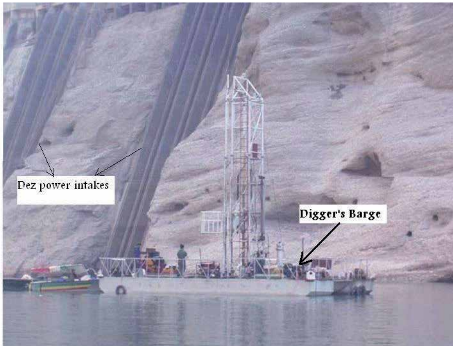
Fig. 3. Photos of barge and digger located near Dez power intakes.
