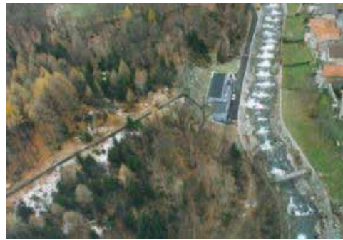
Photo 6. Rino: a view of the power station.
