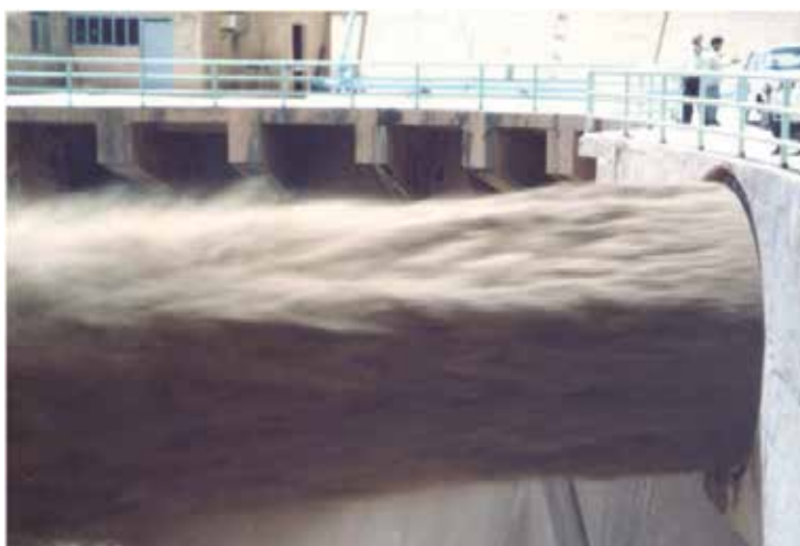
Fig. 9. Photo of Dez Dam Irrigation Outlet, Flushing in June 17, 2003.
