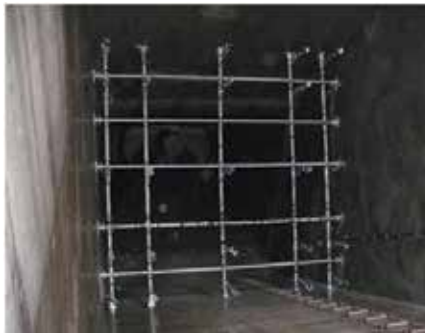
Fig. 14. Hydrometric section with the supporting frame and installed current-meters (own application).
