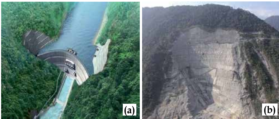
Fig. 12. Geomorphic photograph of the dam site: (a) The layout of key water control, and (b) The right bank slope after excavation.
