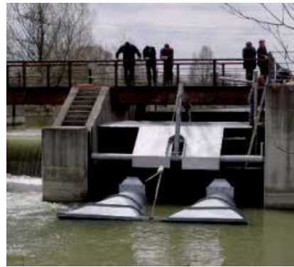
Photo 4. Marchfeldkanal: the turbines.
