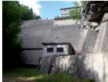
Photo 16. Le Day: The foot of the dam where the small power plant will be set.
