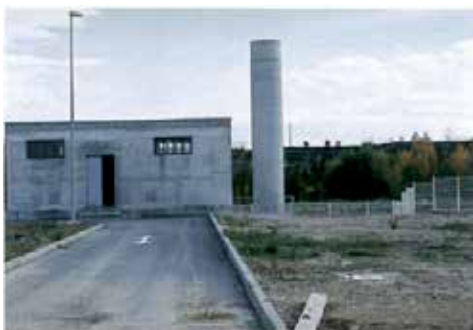
Photo 23. Sangüesa: the biomass plant and its tower of 10.5 meters.
