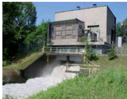
Photo 24. Skawina: the powerhouse during turbine overhaul.
