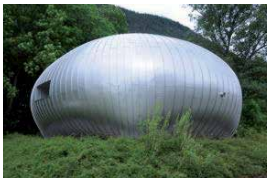
Photo 9. Seefeld: the power house.
