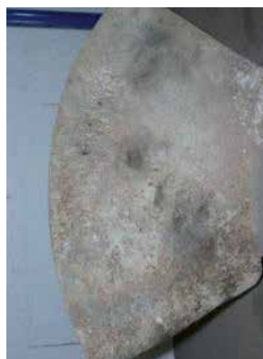
Photo 36. A Kaplan turbine blade, manufactured without hydraulic laboratory techniques, eroded by cavitation after a few months operation.
