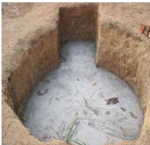
Fig. 10. Concrete bottom of a household unit
