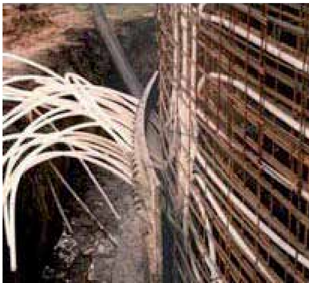
Fig. 13. Integrating the heating tubes (BIOGAS NORD GmbH)
