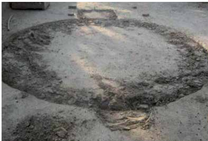
Fig. 5. Marking of dimensions for a biodigester
