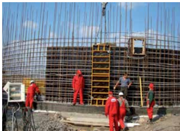
Fig. 11. Building the digester wall for a commercial biogas plant
