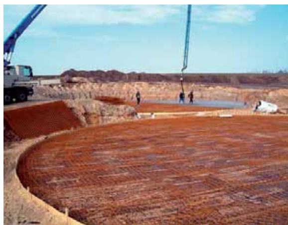
Fig. 8. Structuring the grid irons for a commercial biogas plant (MT-ENERGIE GmbH & Co. KG)
