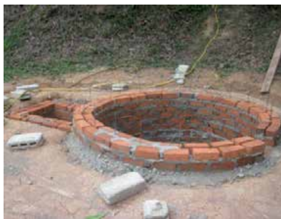
Fig. 12. Building the digester wall of a household unit using burnt-clay bricks
