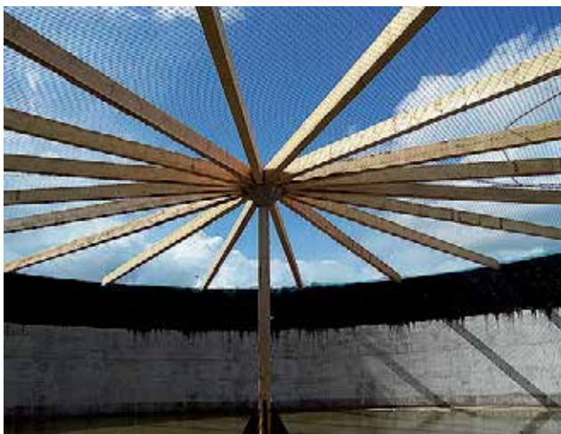
Fig. 14. Wood structure and mesh network that supports the gas holder of digester in a commercial biogas plant (MT-ENERGIE GmbH & Co. KG)
