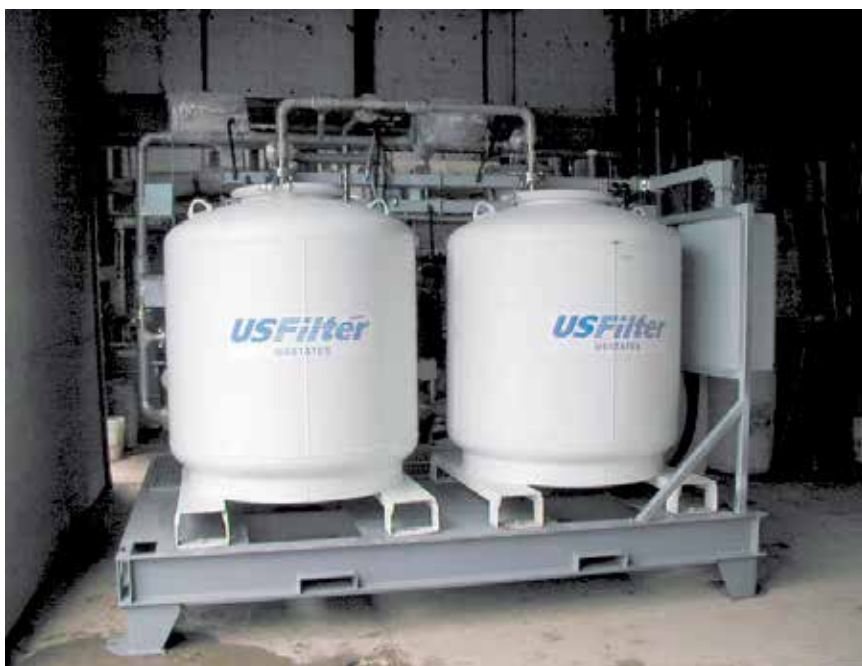
Fig. 19. Activated carbon beds of the GPU (Chandrasekar, 2006)
