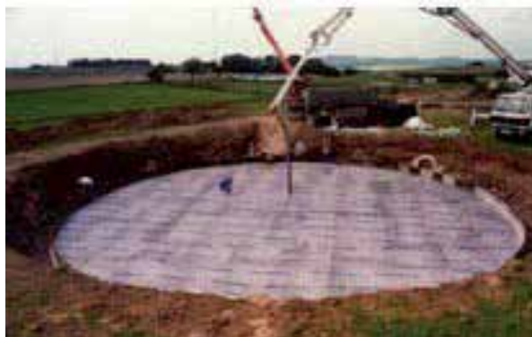
Fig. 9. Pouring the concrete mixture for a commercial biogas plant (BIOGAS NORD GmbH)
