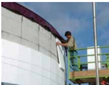
Fig. 17. Installing the insulation (BIOGAS NORD GmbH)
