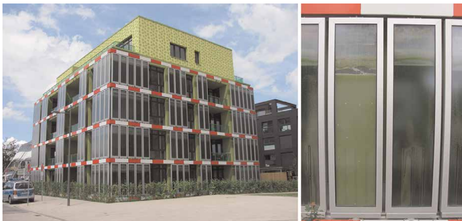
Figure 8. SolarLeaf bioreactor installed in the BIQ House in Hamburg (2013, Arup and Splitterwerk Architects).
