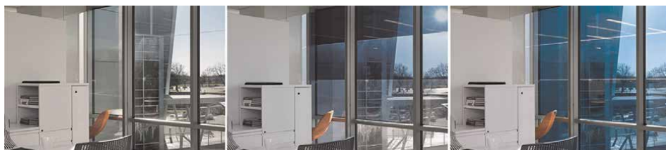
Figure 6. Transition phase in a thermochromic glazed façade.
