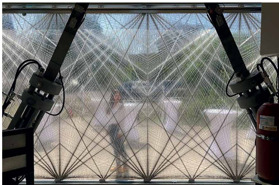
Figure 8. View through the SW fixed panel from inside D1244 © M. Jeong/ILEK.
