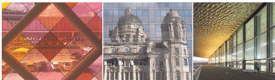
Figure 5. From left to right: tinted glass at Miami International Airport; reflective glass at Mann Island Development Building; selective glass at the Blue Pavilion, Fiera del Mare, Genova.
