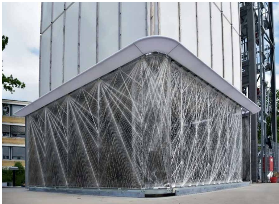
Figure 7. View of FiberSKIN at the south corner of D1244 © M. Jeong/ILEK.
