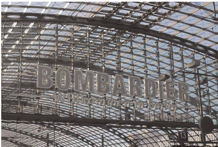
Figure 7. The Hauptbahnhof, Berlin (Germany): Detail of the 1700 m 2 curved surface covered with 780 semi-transparent c-Si panels (Energy output: 180 kWp, Architect: Meinhard von Gerkan; System provider: Optisol, 2003).
