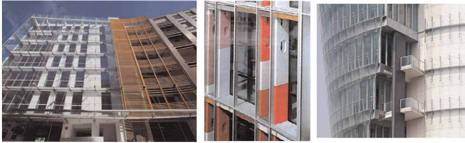
Figure 4. Different types of double glass skin. From left to right: full height, corridors, cells.
