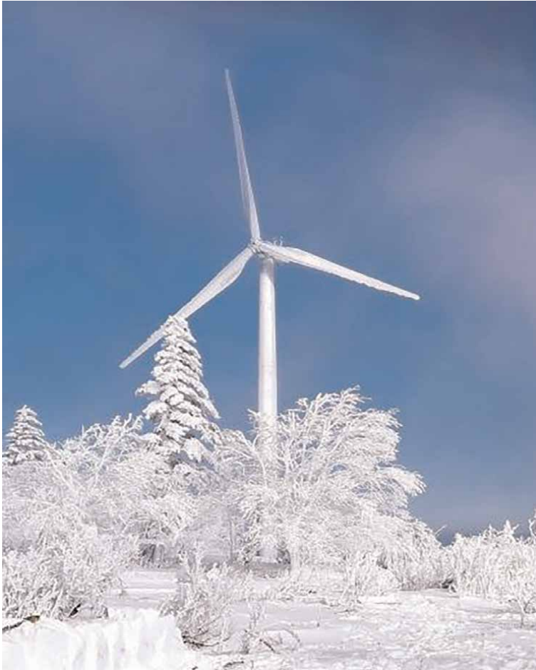
Figure 1. An example of icing on wind turbines.
