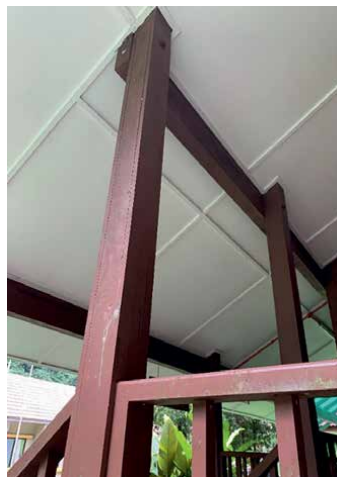
Figure 16. The beams and poles of a house made from Acacia mangium laminated timber.
