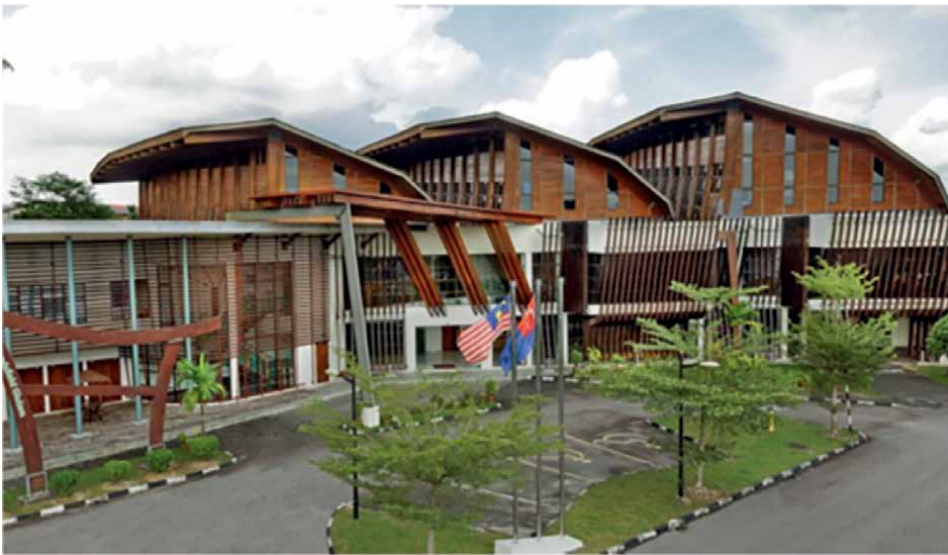
Figure 21. A timber glue-laminated gallery structure in Johore Bahru, Malaysia.
