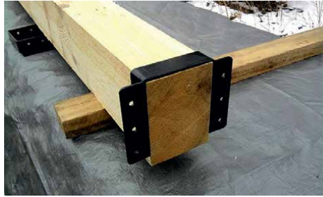
Figure 10. Another design of the universal end joint braces.
