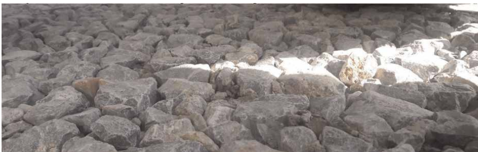
Figure 25. The ballast particles placement under the sleeper in RRP 235special method.
